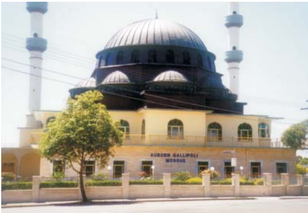
Auburn Gallipoli Mosque, Sydney, Australia
